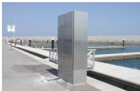
➔ Stainless steel 1200amp electrical panel.
