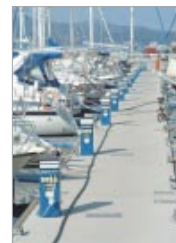
➤ Computer controlled MAXI bollards
