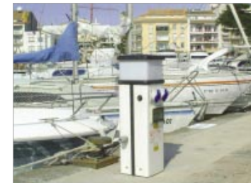
➤ 500mm Foamex bollard with two 16 amp sockets and two direct connection water outlets.
